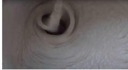
2 Mix Skamol Structural Plaster with water according to the specified mixing ratio.
