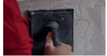
3 Apply Skamol Structural Plaster at an even layer thickness of 2 to 8mm.
