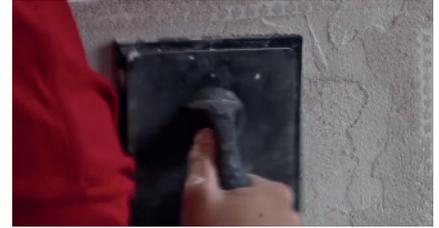
**3** Apply Skamol Smooth Plaster in an even layer thickness of 1.5 to 3mm.
