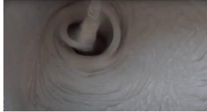
**2** Mix Skamol Smooth Plaster with water according to the stated mixing ratio.
